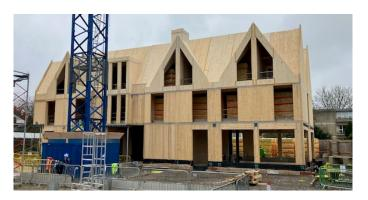
The construction of the cross laminated timber frame for the next building will start in early April and will mirror the frame just completed. It will be erected using Sparkle our tower crane. As before the pre-manufactured bathroom pods will be positioned as the timber panels are erected.
