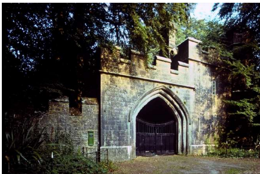
UC:P351/3/P1/25: County Cork, Castletownroche, Annes Grove, the castellated gate-lodge, designed by Ireland's only Pre-Raphaelite architect, Benjamin Woodward, and built in 1854 to give access to the Dublin road, 1984.
