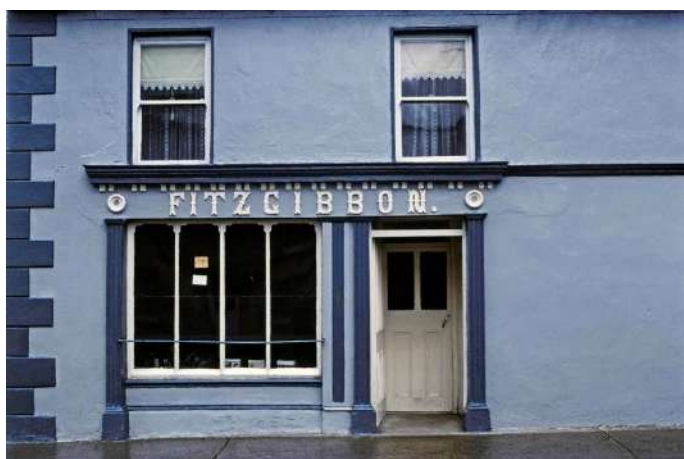
UC:P351/3/P1/158: County Tipperary, Fitzgibbon shop front, 1982.
